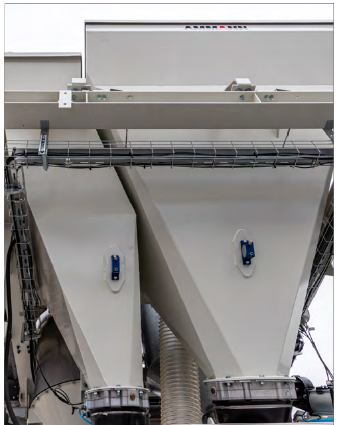
Weighing platform with cement weigher and optional silica weigher.
