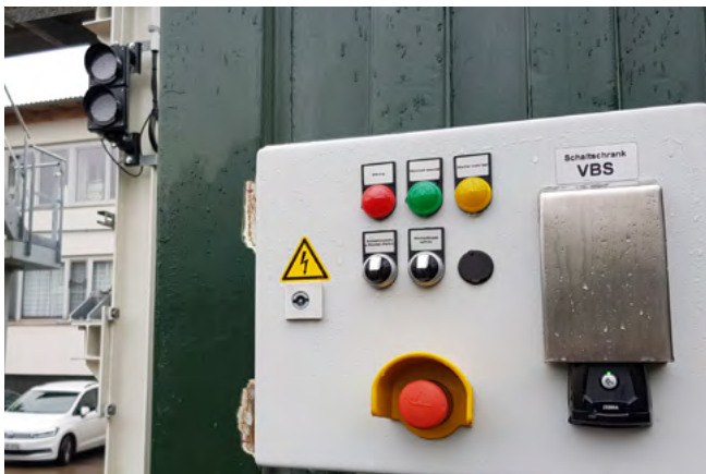
Option: Barcode scanner and traffic light system (concrete filling station).
