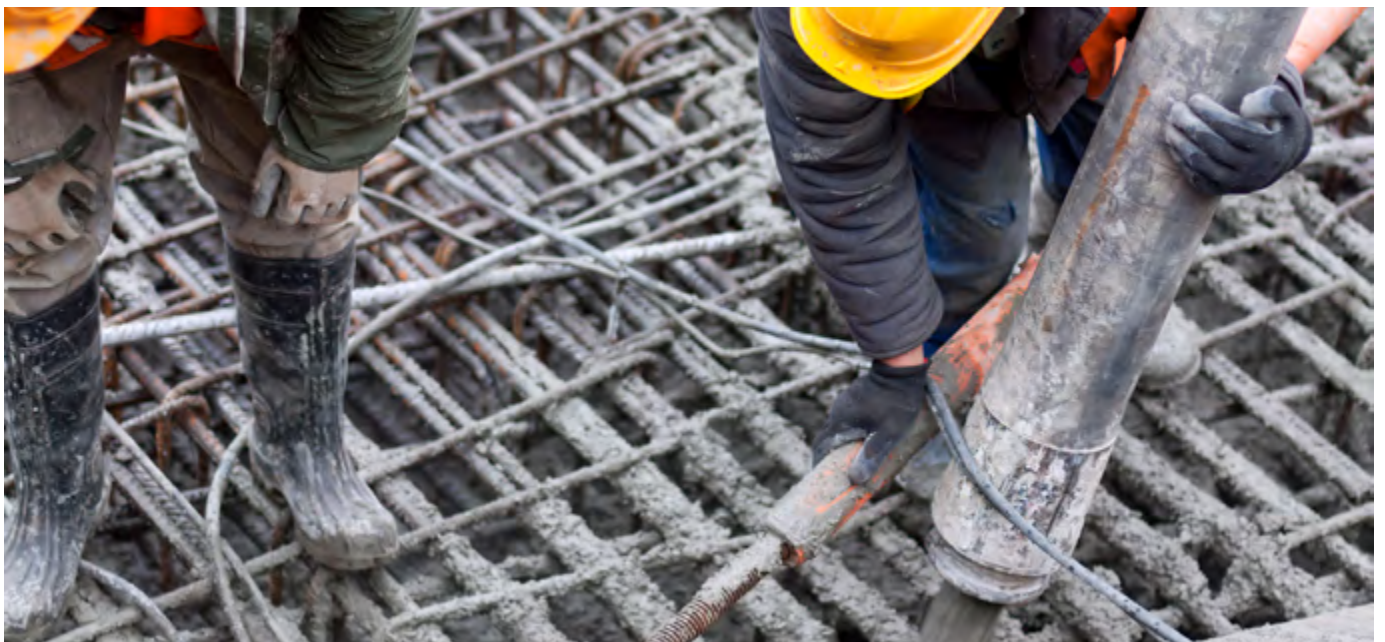
Typical installation of ready-mix concrete.
